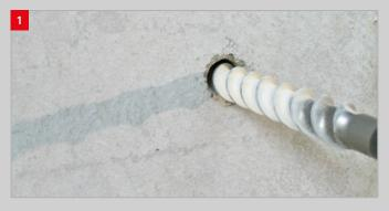
Drill a **25 mm-diameter hole** with an impact drill and masonry drill. If necessary, rework the core drilling on the outer wall.
