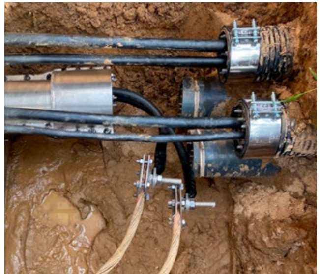
GPD-CV93/G/60/WE50/V2A/EPDM/ (Z)x(D): for sealing exposed corrugated pipes
